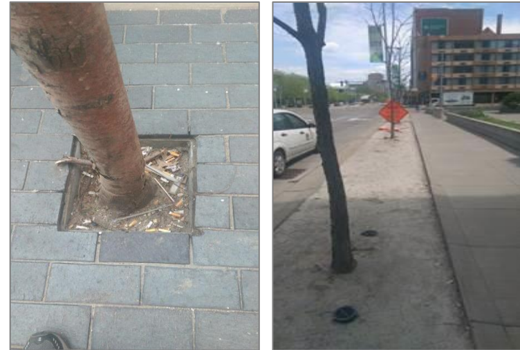
Left: Without clear planting specifications in place, investment is wasted and there is little recourse to replace trees. Trees planted by contractors as part of a casino project lack adequate planting space. Right: Trees are planted by contractors in such poor soil that even weeds will not grow.
