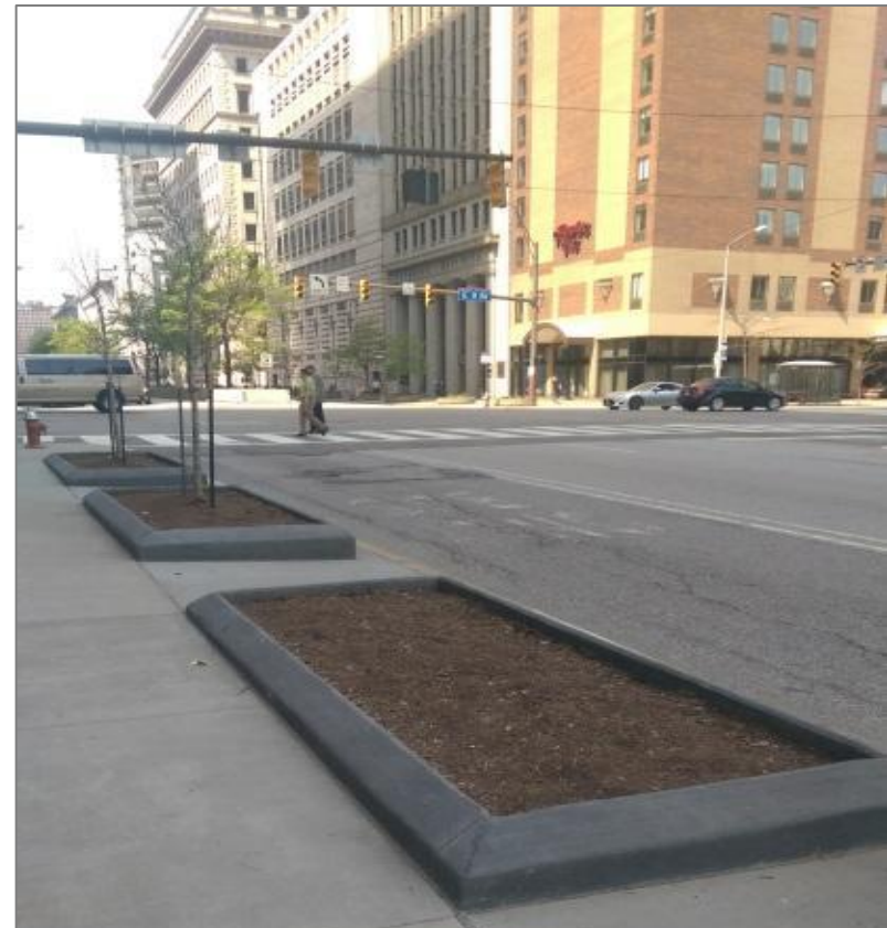
A tree is missing from a newly constructed tree pit on East 9 th . With a strong ordinance and penalty structure in place, parties can be held responsible to replace missing trees. Image courtesy of City of Cleveland.
