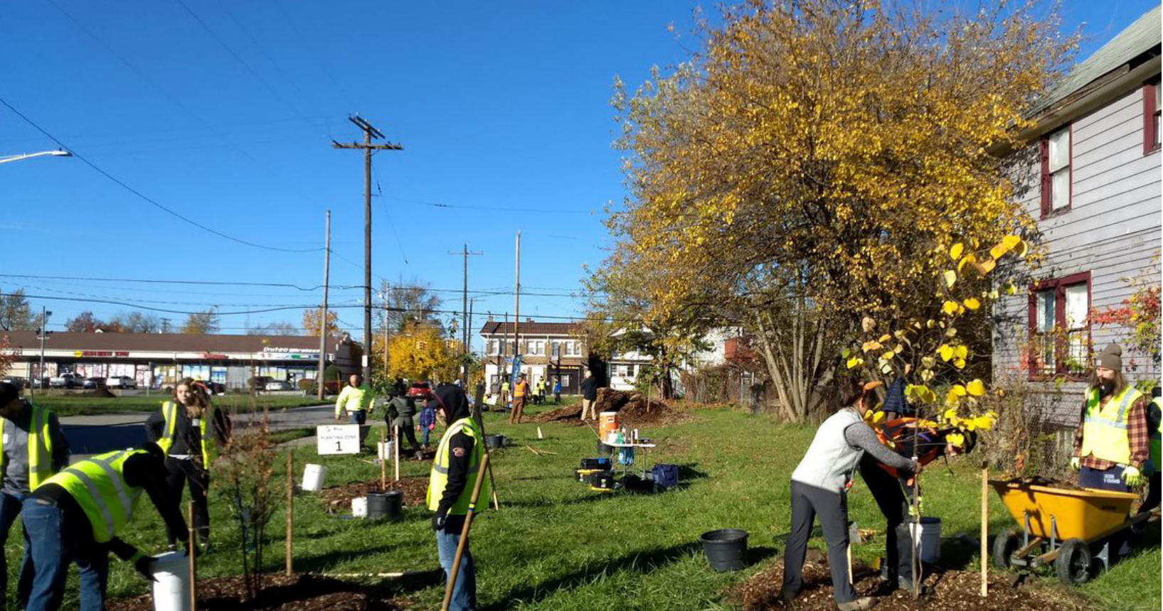
GREEN DEVELOPMENT will reduce maintenance burden, increase quality of life, and climate resiliency.
