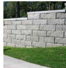
OPTIONAL RETAINING WALL RECON WALL SYSTEMS - CONCRETE
